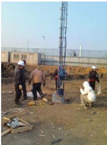
Installing the O-cell
