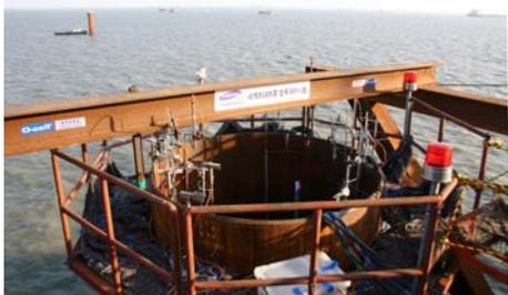
*Top of pile instrumentation and reference
