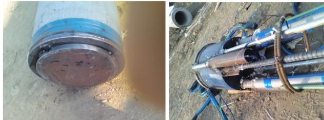
Prior to driving the first section of pile, a special shoe was inserted into the hollow section of the PHC pile and welded in place. The shoe acts like the plug of soil that forms inside the PHC pile during open-ended driving conditions but also allows for a suitable bearing surface for the base of the O-cell. The O-cell, related instrumentation and strain gauges already fixed to a reinforcing cage were inserted into the hollow centre of the PHC pile and concreted in place.
