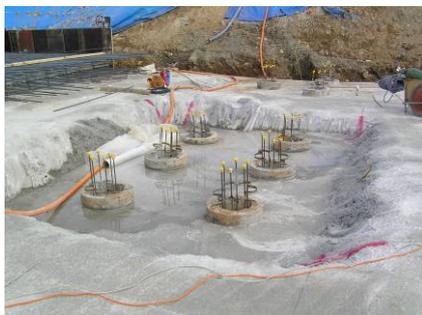
As the O-cell test was conducted on a production pile, after completion of testing, the O-cell and annulus surrounding the O-cell were grouted by the foundation contractor to restore structural integrity to the pile and the pile element was incorporated into the works.
