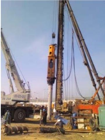
Driving the PHC Test Pile
