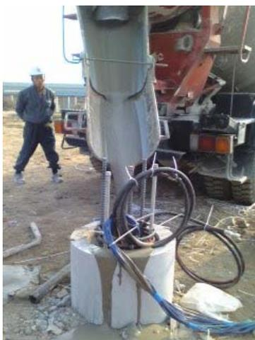
Concreting the PHC pile
