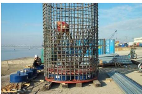
Final assembly of reinforcing cage with O-cells
