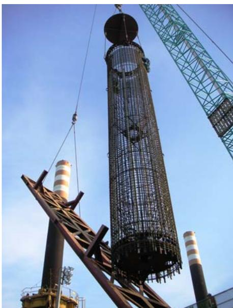
*Bottom Cage being prepared for insertion into
