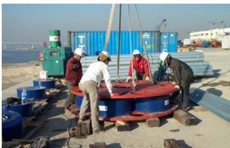
Assembly of the bearing plates for the O-cell arrangement
